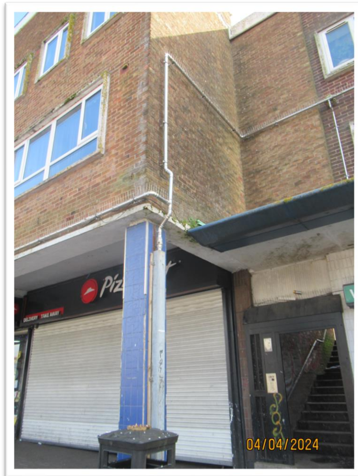
Figure 27: Countisbury Avenue MOB after replacement (new vertical)
