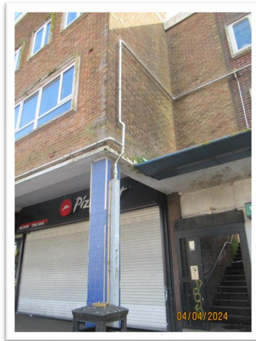
Figure 11b: Countisbury Avenue MOB after replacement (new vertical)
