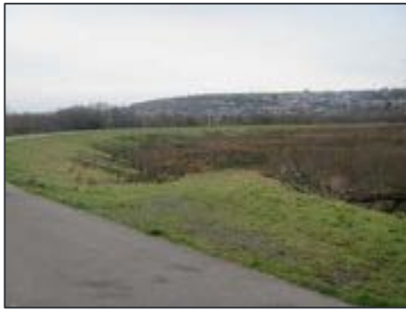
Flood embankment looking south west
