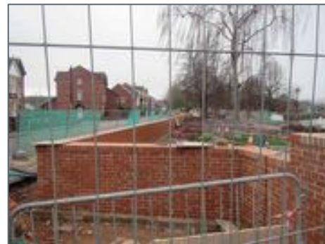
Environment Agency flood wall construction
