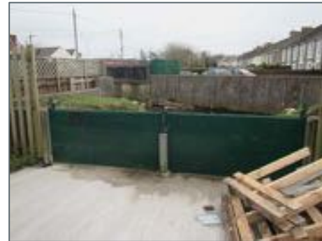
Removable flood barrier on right bank of river near Location A
